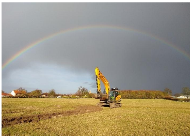
Figure 1: Excavator at work
